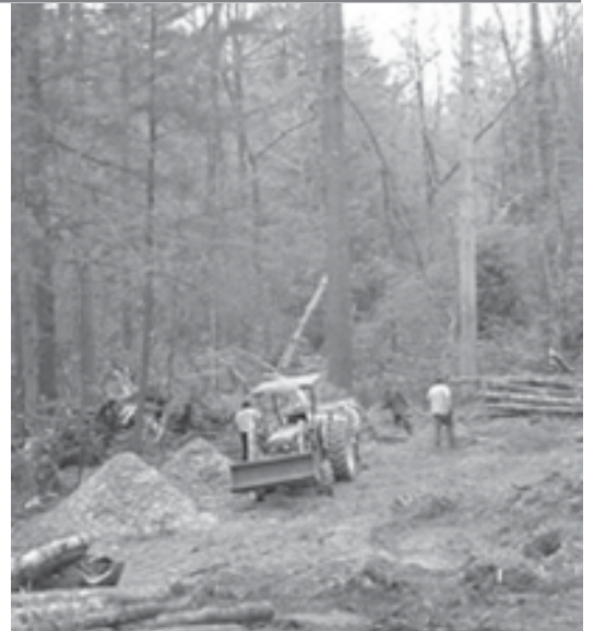
New Parking created adjoining house
